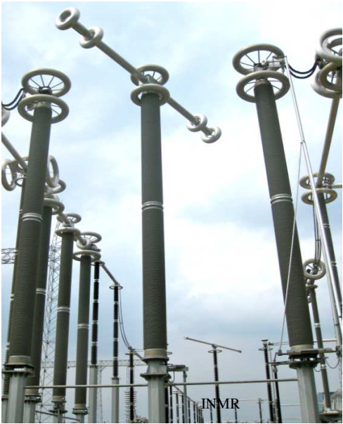
Fig. 4 Bypass Disconnector for the world's first commercial 800kV DC transmission system energized in December 2009.
