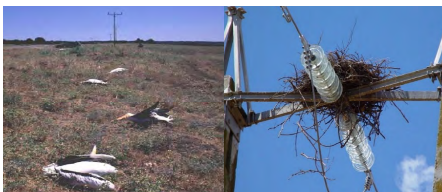
Figure 6. Pelicans dead from clashing conductors, Israel and nest likely to cause flashover, Spain.
