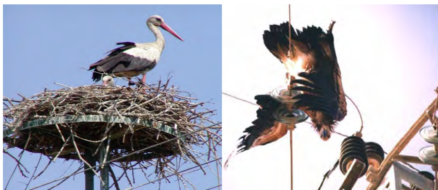
Figure 5. Migratory stork nest in Greece and griffon vulture fatally bridging in Israel.
